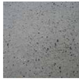
General Polished Concrete
